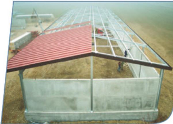
Structures made with beams through the classical Buton-Tirant technique.
