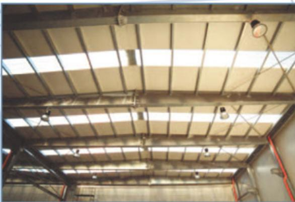
The internal white refinishing, eventually combined with skylights or windows make the inside much brighter, still complying with specific regulations
