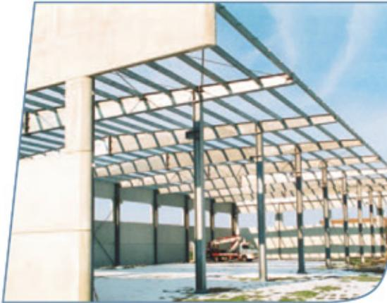
Solid/core beams assembled with tubular elements.
